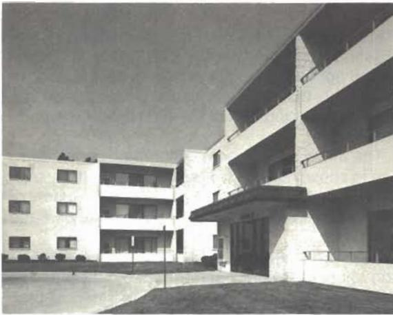
Many firesafety-conscious communities are insisting upon fire-resistant construction for low-rise apartment buildings. The concrete floors and masonry in this building resist fire, reduce property loss, and protect residents. (Photo © Thom Abel 1978)
