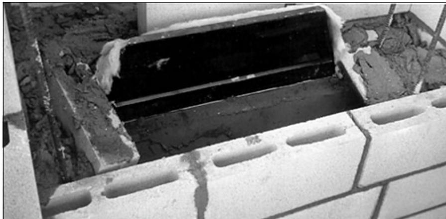
**Figure 3-6** Construction of masonry fireplace showing installation of damper.
